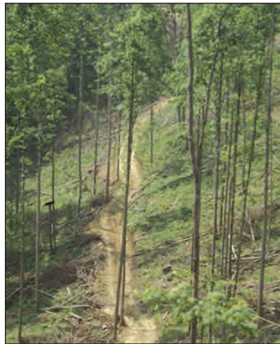
Figure 9.17. Skid trail placed with curves or turns where water can easily run off the surface.
