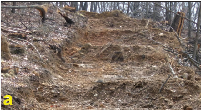
Figure 7.13. Practices to implement inside of minimum SMZ distances include increased frequency of water control structures (a), or properly placed debris directly below water control structures to reduce runoff reaching streams (b).
