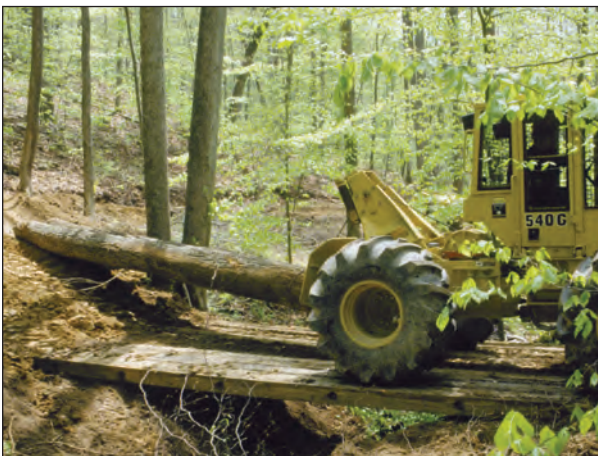
Figure 8.2. Wooden skidder bridge with bumper trees to assist in keeping loads behind the skidder while crossing the bridge.
