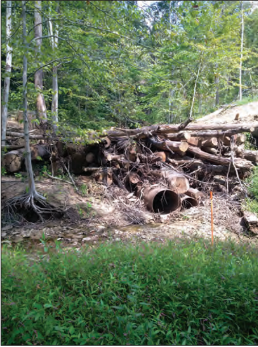
A high-traffic primary skid trail approaching a landing using steel pipe backfilled with poles to minimize soil in the channel.
