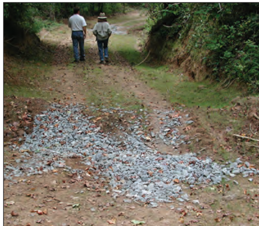
Figure 12.9. A small reserve grade structure with gravel on a retired haul road. The size, with the addition of gravel, is sufficient to handle light traffic by the landowner.
