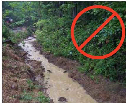
Figure 9.2. To reduce mud on the landing, soil was pushed into a small headwater stream.
