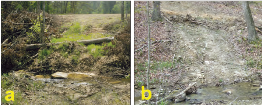
Figure 12.13. Crossing was removed and fill soil was back dragged from the stream and seeded (a). Water control structure was placed directly above the approach so that runoff from skid trail did not wind up in the stream (b).
