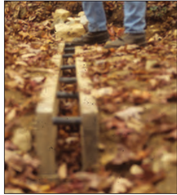
Figure 12.10. Box culvert used on retired and compacted haul road.
