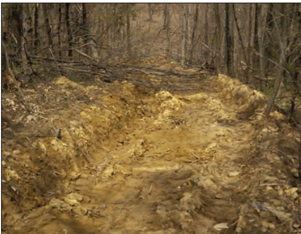
Figure 9.18. A rutted skid trail typical of operations during wet weather, requiring attention if runoff can potentially reach a stream or channel.
