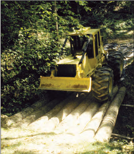
Figure 8.5. Log bridge developed using recommended lashing design.
