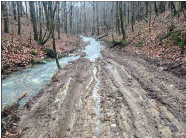
Figure 7.5. Equipment operations in streams can cause pollution and directly impact aquatic species.
