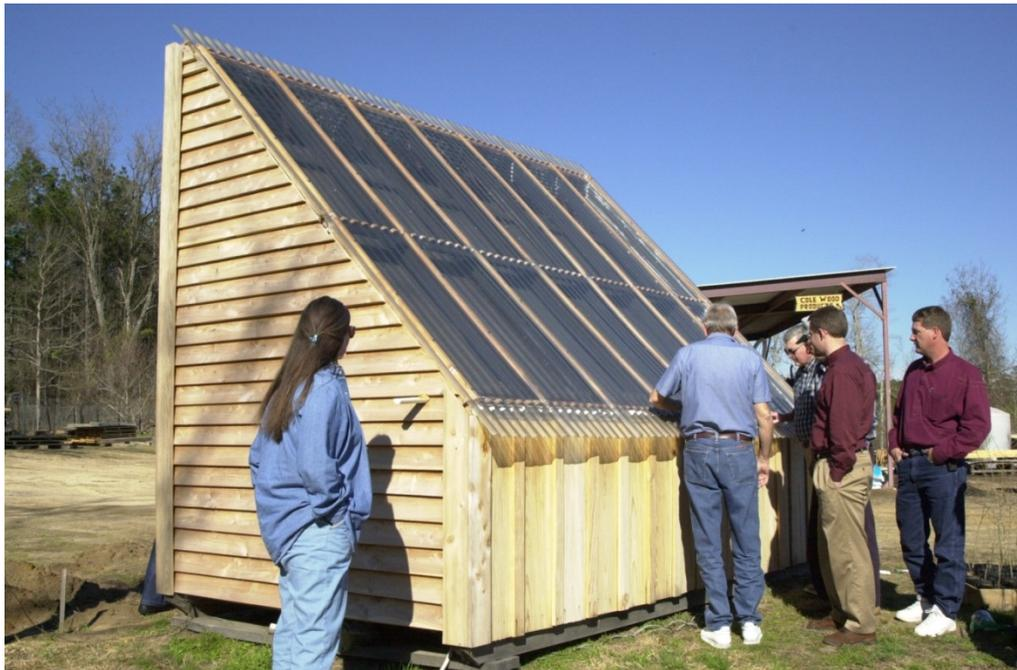
**Figure 6.** Solar dry kiln. The sloped roof acts as a solar collector to heat the dry kiln.
