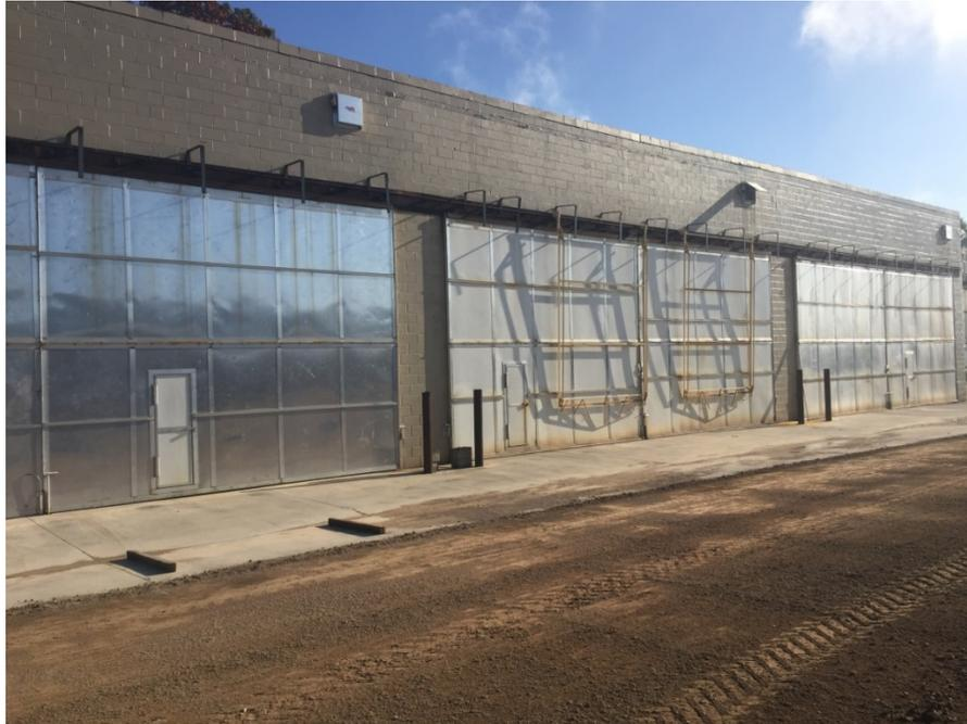
**Figure 5.** *These are dehumidification kilns, though it's hard to tell the difference from most other kiln types just by looking at the outside of the building. One difference from large conventional kilns is that the vents are smaller and fewer in number (in this photograph the vents are above the doors at the front of the building). Each of these large kilns holds about 50,000 board feet of lumber.*
