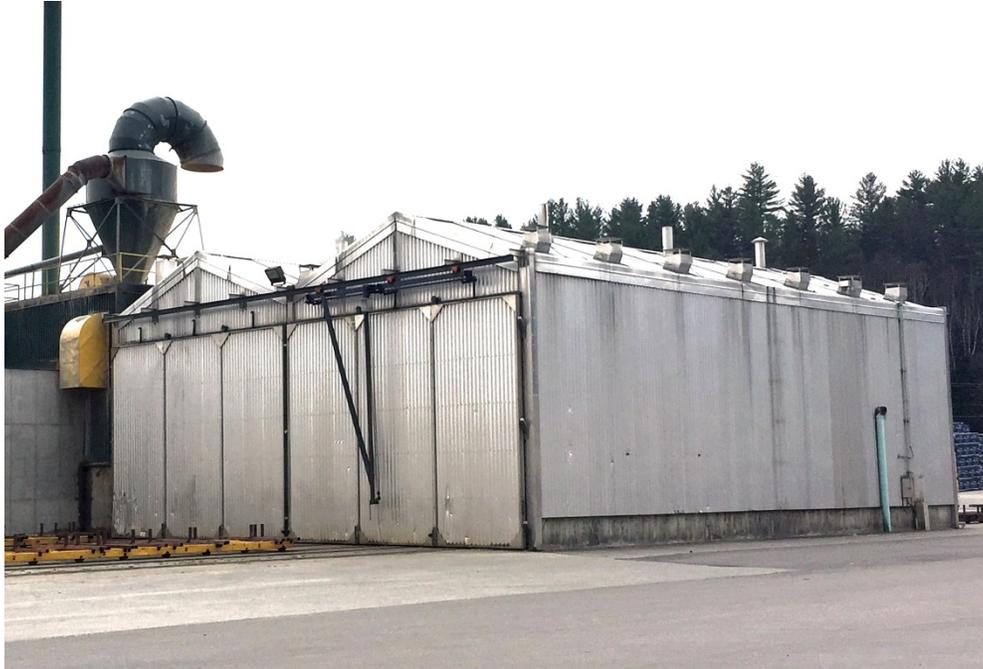
**Figure 1.** Conventional steam-heated dry kilns. There are large doors for loading the lumber in the front of the kiln, and the kiln is constructed from corrosion-resistant materials. Notice the number of vents in the kiln roof. These are used to vent water vapor from the drying lumber.
