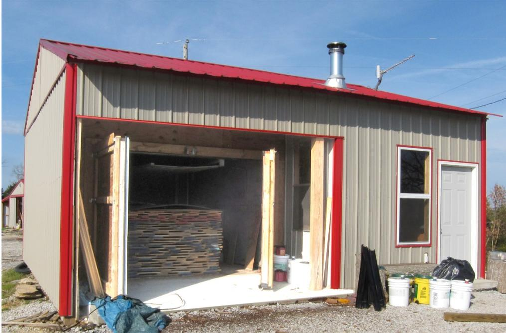
**Figure 3.** The DH kiln at the left holds 4000 board feet of lumber. The door at the right is for access to the office, all under one roof at this small company. The stove pipe serves as a chimney for a small wood-fired box stove used to heat the office. This kiln was designed with a narrow door and the lumber has to be loaded sideways.
