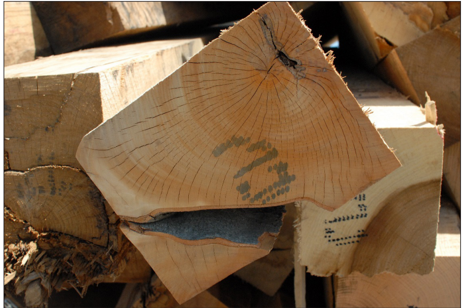
Figure 18. This beech bark seam is essentially a split and can't be saved with an end plate.
