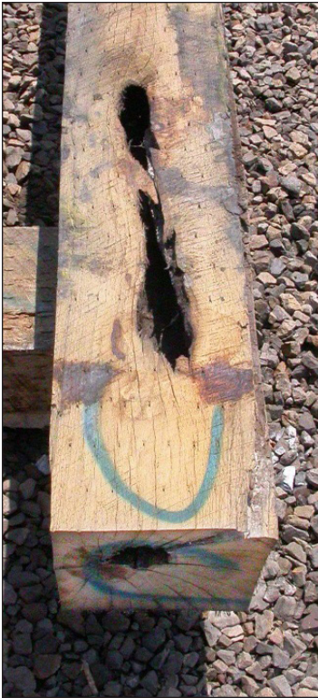
Figure 11. Large holes caused this tie to be culled. Notice how the hole extends from the end of the tie into the RBA.
