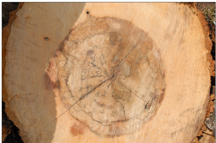
Figure 17. Log with split. If this split doesn't widen too much when the log is cut, it would probably be plated with a gang nail plate and could make an excellent tie.
