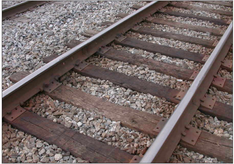
Figure 1. Section of railroad track used to move freight through Lexington, Kentucky. This track uses wooden crossties.
