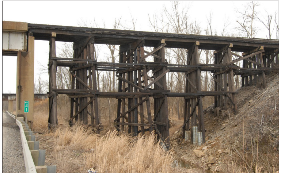
Figure 4. Wooden trestle bridge across the Pennyrite Parkway near Madisonville, Kentucky.
